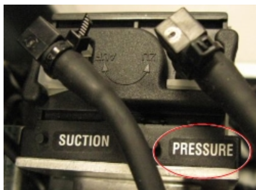
Figure 6-126 Tubes connected to the waste pump
